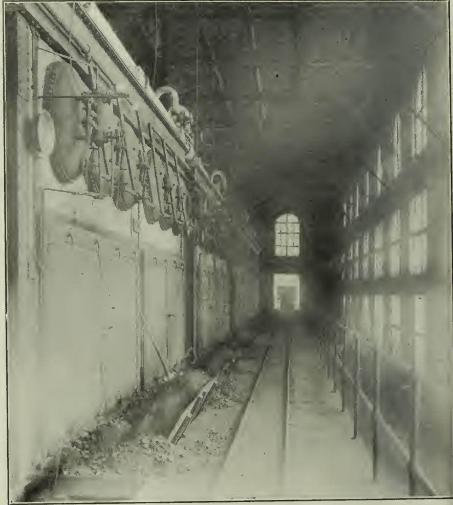
FIG. 5. METHOD OF HANDLING COAL IN BOILER ROOM.
